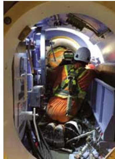
Divers entering the working chamber from a TBM air lock.
